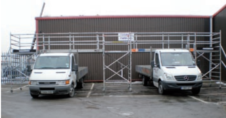
Bespoke Tower Scaffold
