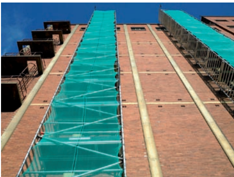
Octo 250 Tower Scaffold
