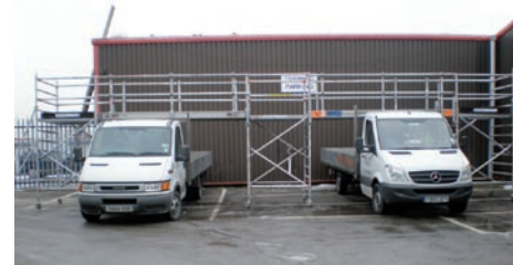
Bespoke Tower Scaffold
