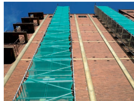
Octo 250 Tower Scaffold
