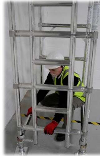
3. From inside the tower, fit in 2 horizontal braces to the vertical member of the frames, as low as possible, below the 1<sup>st</sup> rung.
