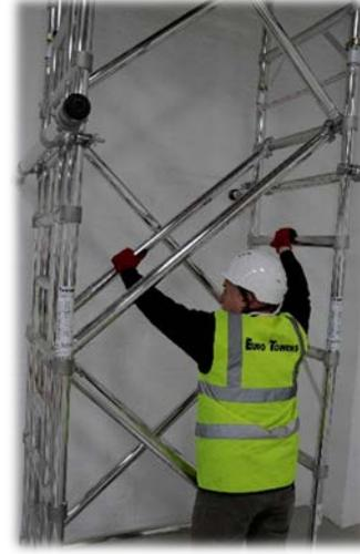
15. ALL TOWERS ABOVE 10.69m PLATFORM HEIGHT DOUBLE BRACE THE BASE THEN REPEAT STEPS 8 – 12. Fit 4 diagonals to the 2 base run of braces running in opposite directions to the existing ones on the tower. You should create an X on each side on the first 2 levels of braces
