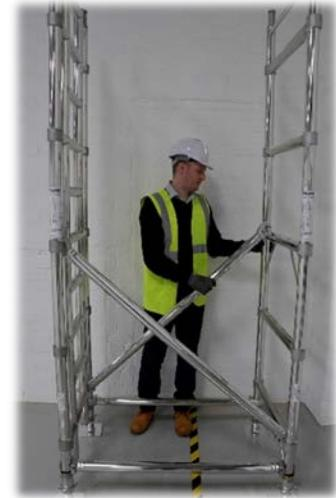
4. Add 2 diagonal braces from the 1st to 3rd rungs as shown, check and adjust the base position (if required) for the build.
