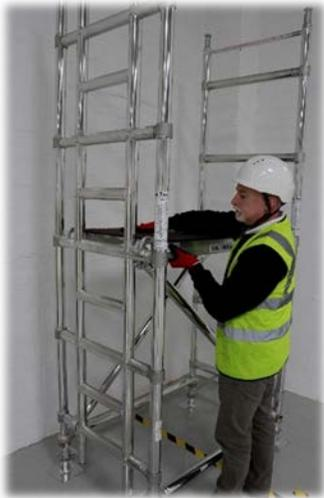
5. Add temporary trapdoor platform to the 3rd rung, trapdoor at the ladder end.
