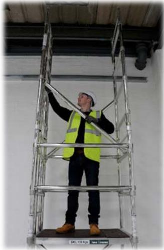
9. Fit 2 diagonals to the frame rungs in a cross pattern starting 2 rungs up from the platform. ALL other platform levels start 1 rung up from the platform.
