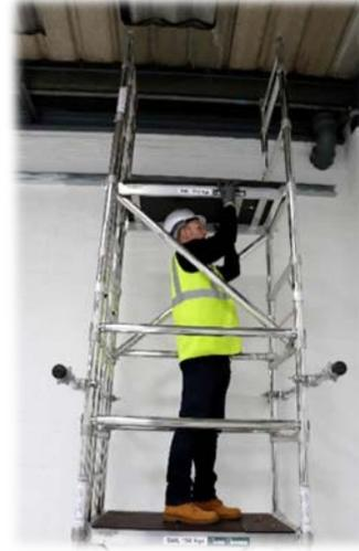
11. Fit the next trapdoor platform to the 4<sup>th</sup> rung above the platform alongside the brace hooks. Ensure the trapdoor is at the ladder end,
