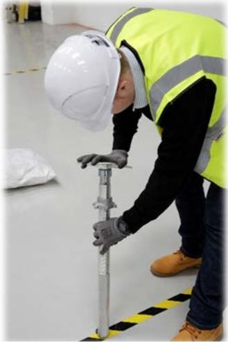
1. Insert a base plate into each adjustable leg, leave approximately 25mm between the nut and the end of the leg for levelling purposes.
