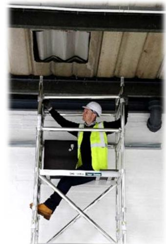
12. Sitting through the trapdoor fit 4 horizontal braces to the verticals above each rung of the frames above the platform to complete a guardrail.
