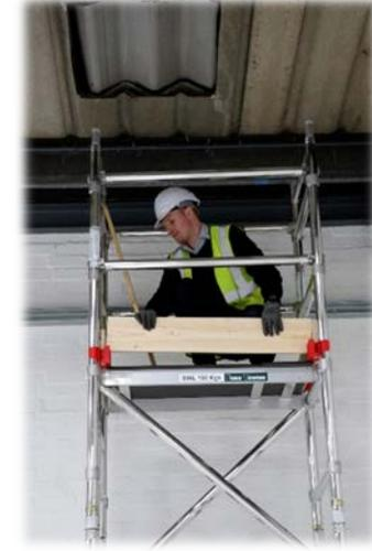
16. Fit toeboard clips and toeboards to complete the tower.
