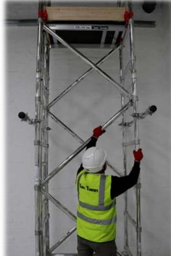
14. Fit 2 diagonal braces to complete the brace run on the tower. THIS COMPLETES THE BASE SET UP FOR ALL TOWERS UP TO 10.69m PLATFORM HEIGHTS. REPEAT STEPS 8 - 12 UNTIL YOU REACH YOUR REQUIRED HEIGHT. GO TO STEP 16.
