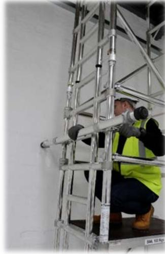
10. Fit a side prop to the outside of the frames at each end above the platform ensuring the couplers are tight, wind the legs to engage the walls, check there's no side movement. FIT SIDE PROPS EVERY OTHER PLATFORM LEVEL.
