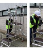
Add the additional brace below the platform. For a stepfold 2 you should now the ribbed brace. Then have 2 ribbed braces below the working platform.
