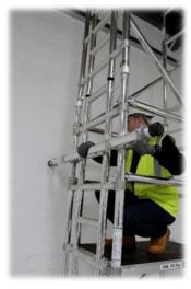
10. Fit a side prop to the outside of the frames at each end above the platform ensuring the couplers are tight, wind the legs to engage the walls, check there's no side movement. FIT SIDE PROPS EVERY OTHER PLATFORM LEVEL.
