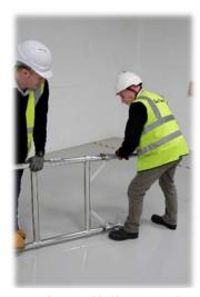
2. Insert the assembled legs into each 5 rung frame.
