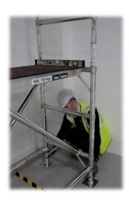
6. Level the tower adjusting the leg nut using a spirit level as a guide.
