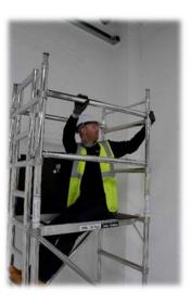
7. Sitting through the trapdoor fit 4 horizontal braces to the verticals above each rung of the frames above the platform to complete a guardrail.
