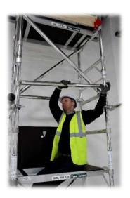
13. Go back down to the 1st platform, sitting through the trapdoor remove all the guardrail braces and descend to the ground and remove the temporary platform.
