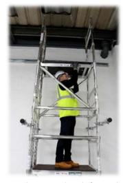
11. Fit the next trapdoor platform to the 4<sup>th</sup> rung above the platform alongside the brace hooks. Ensure the trapdoor is at the ladder end,
