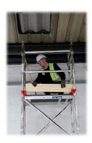
16. Fit toeboard clips and toeboards to complete the tower.
