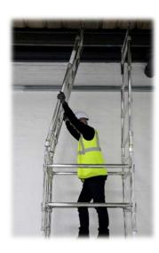
8. Fit a 4 rung ladder and 4 rung plain frame to the 5 rung base frames, ladders MUST run continuously throughout the tower; lock in place with the interlock clips.
