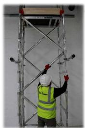
14. Fit 2 diagonal braces to complete the brace run on the tower.
