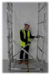
4. Add 2 diagonal braces from the 1st to 3rd rungs as shown, check and adjust the base position (if required) for the build.
