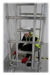
3. From inside the tower, fit in 2 horizontal braces to the vertical member of the frames, as low as possible, below the 1st rung.
