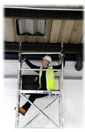
12. Sitting through the trapdoor fit 4 horizontal braces to the verticals above each rung of the frames above the platform to complete a guardrail.
