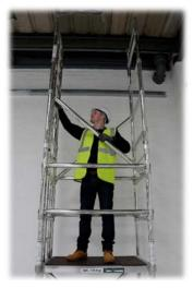
Fit 2 diagonals to the frame rungs in a cross pattern starting 2 rungs up from the platform. ALL other platform levels start 1 rung up from the platform.
